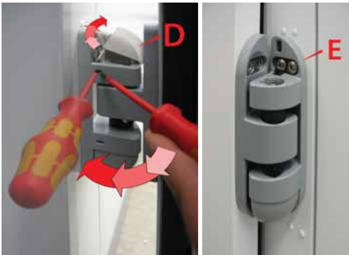
Pic. serie 13. Assembly of the hinges
