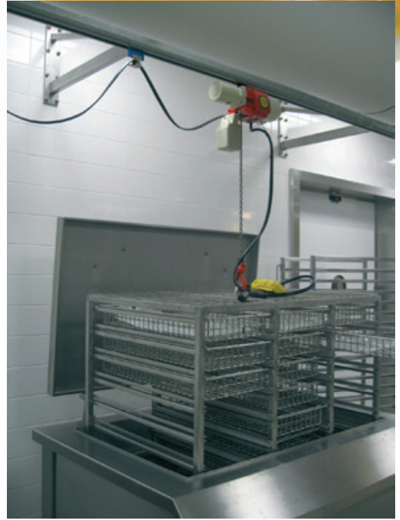
Rail system for lifting baskets
